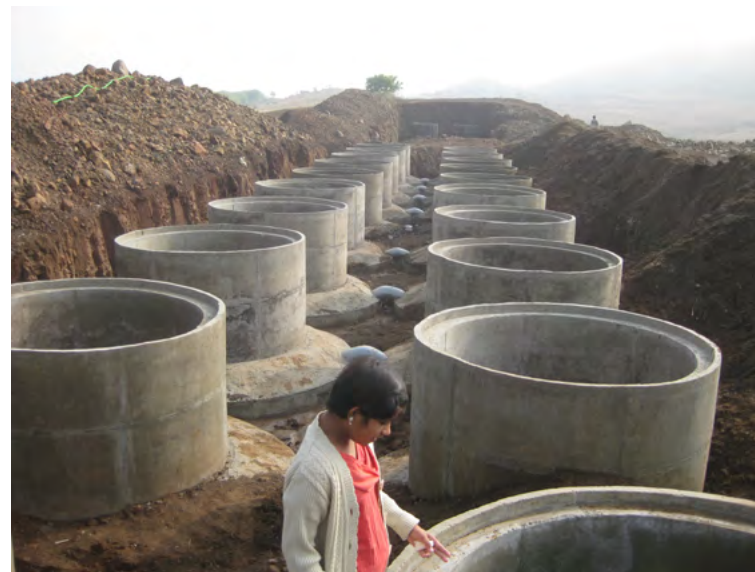
Community biogas system being constructed at Payvahir
